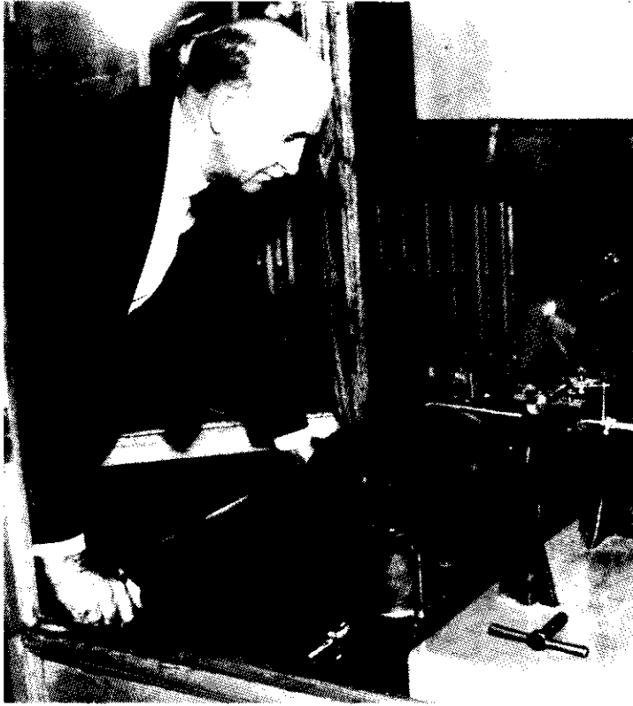
Fig. 3-3. Dr. Frederick J. Pack inspecting recording drum of Bosch-Omori seismograph (ca. 1930?).
