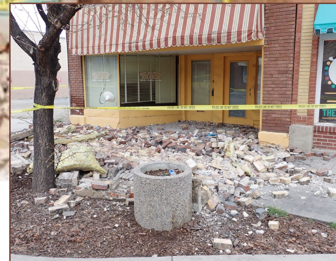
Top: Structural damage to a store in downtown Magna caused by the M5.7 Magna earthquake. Strong ground shaking caused part of a brick wall to collapse. Photo courtesy of Utah Geological Survey.
