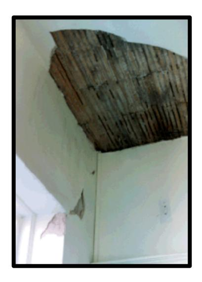
Plaster damage occurred in the women's restroom in the St. George Art Center in St. George, Utah. This building is a large, two-story building constructed of unreinforced masonry.
