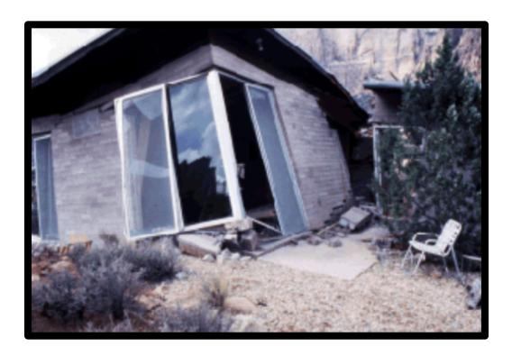
Balanced Rock Hills Subdivision was built on "slide hill" (name given the area by old-timers in the area. The earthquake, whose epicenter was 30 miles away, caused slide hill to slide again. This is one of three homes destroyed in the landsliding. No one was injured. Photo by B.D. Black, Utah Geological Survey.
