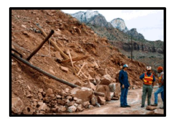
Utility poles along State Route 9 were turned to kindling by the steep bulging front (toe) of the landslide as it moved laterally several meters.
