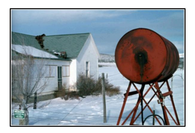
Chimney bricks dropped onto the roof and front porch of this farmhouse located in Pocatello Valley, Idaho.
