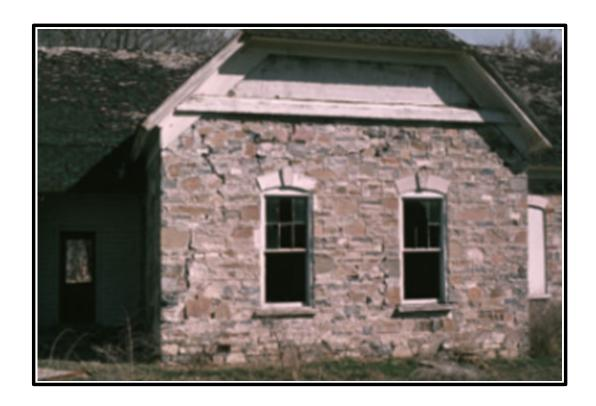
In Snowville, Utah, this stone building was cracked by the ground shaking.
