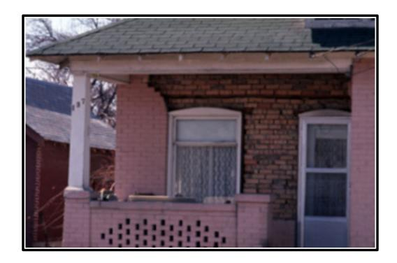
In Malad City, Idaho, the brick facade was stripped off the front wall of the Thorp home and landed on the porch. Inside, irrreplaceable antiques were smashed.
