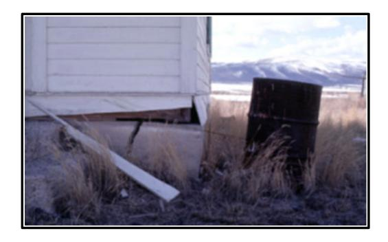
This farmhouse in Ridgedale, Idaho, had its foundation severely cracked during the earthquake.
