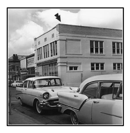
Logan Junior High School was severely damaged by the earthquake, but was repaired and allowed to reopen within two weeks. A reinforced concrete bond beam was cast around the walls at the roof line, and steel tie rods were installed. Structural engineers reported that this work would make the school more safe than it was before the earthquake. This photo shows the brick replacing the original loosened parapet wall.
