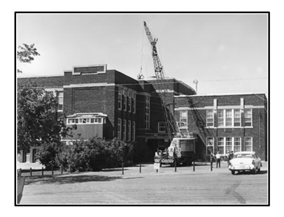
At North Cache High School in Richmond, Utah, cranes are used to remove the heavy (150 pounds per square foot) capstones that were loosened during the earthquake.
