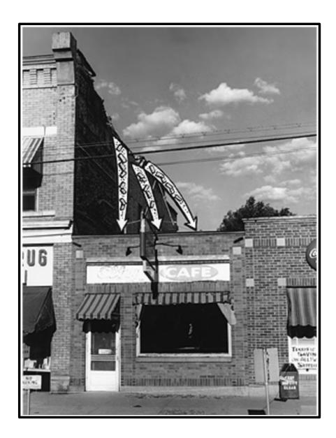
Arrows show path of bricks that tumbled from the parapet of the Lewiston Drugstore onto the roof of the City Cafe in Lewiston, Utah. Luckily this cafe in Lewiston, Utah, was not open when ground shaking caused part of a brick parapet of an adjacent building to fall through the roof. Photo by Ray G. Jones.
