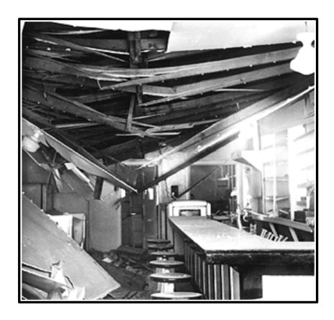
Luckily this cafe in Lewiston, Utah, was not open when ground shaking caused part of a brick parapet of an adjacent building to fall through the roof.
