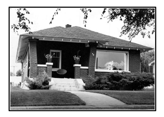
Brick porch columns on this home in Richmond, Utah, were cracked and tilted by the ground shaking.
