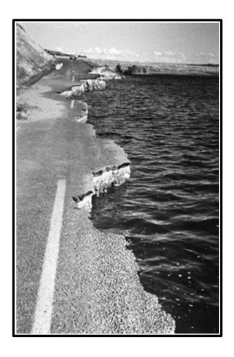
Four small landslides dropped portions of Highway 287 into Hebgen Lake, blocking the exit route for people in the Madison Canyon above the landslide. Photo #116 from I.J. Witkind Collection, U.S. Geological Survey.
