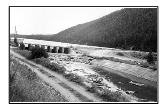
The spillway of Hebgen Dam was damaged by the ground shaking. Water flowing down the spillway further eroded some of the concrete slabs.
