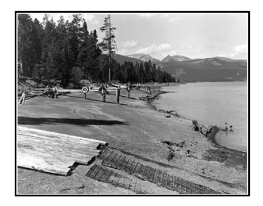
Northward tilting of Hebgen Lake submerged the north shore and left these boat docks high and dry along the south shore. This down-dropping of the lakebed caused the waves that overtopped the dam 4 times and continued oscillating 11 1/2 hours. Photo #53 from I.J. Witkind Collection, U.S. Geological Survey.
