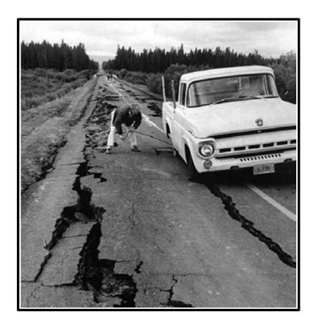
Ground shaking caused roadbeds to settle and crack, hampering safe driving. This highway is U.S. 91 between West Yellowstone and Hebgen Lake. Photo by Ray Jones, Deseret News.
