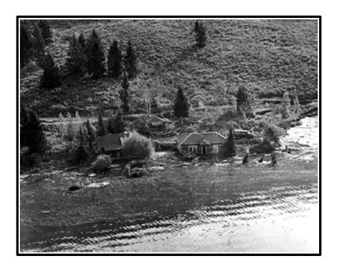
Hebgen Lake surrounded these units of Hilgard Lodge on its northeast shore when the basin beneath the lake dropped (subsided) over a large area during the earthquake.
