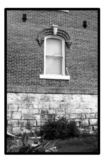
Close-up, taken in 1991, of one wall of the Beaver County Courthouse. Notice the crack beneath the window. The decorative elements are probably each one of a pair of "turnbuckles" on opposite walls connected by heavy wires in a retrofit effort to protect the building from further damage. Photo by Edith O'Brien.
